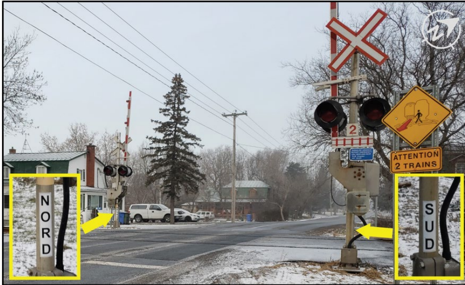
Figure 3. Saint-Féréol Road grade crossing, with inserted images showing the “NORD” and “SUD” stickers (Source: TSB)
