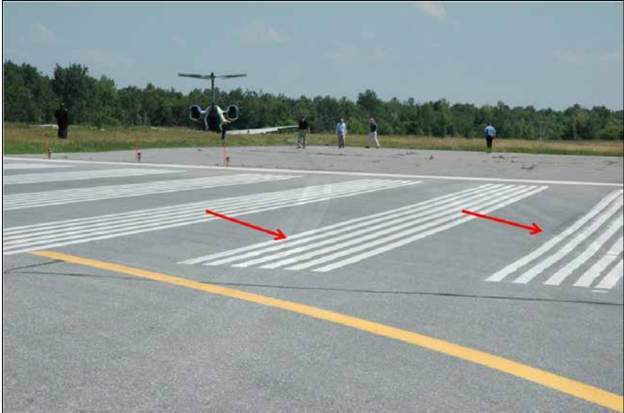
Photo 2. Steam-cleaned marks observed on the departure end of Runway 07
