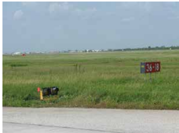
Photo 2. Right runway holding position sign and runway guard lights viewed from Taxiway Victor
