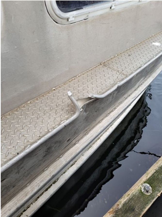
Figure 5. Damage to the vessel's starboard side hull (Source: Vessel owner)
