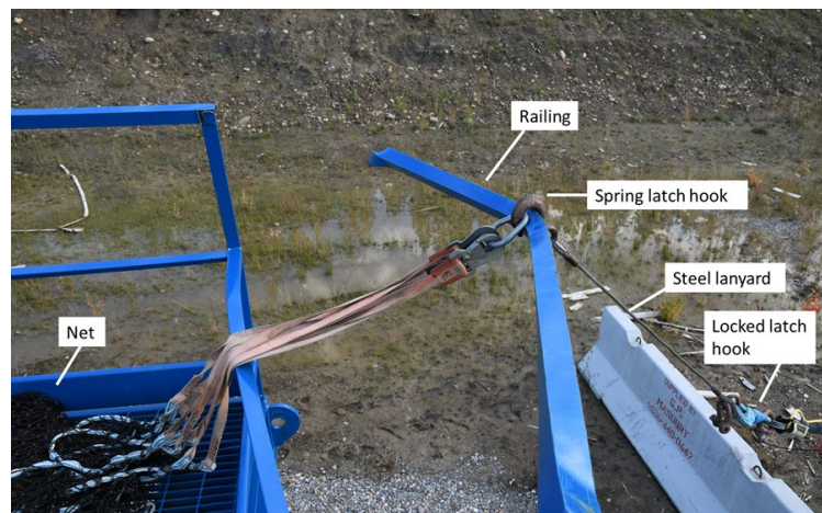
Figure 4. Image of hook and railing (Source: TSB)
