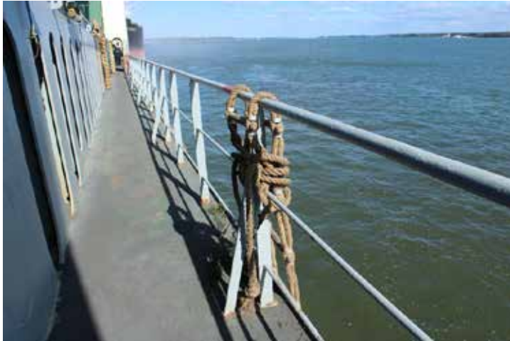
Figure 6. Rigging of Jacob's ladder to the guardrail on the Amazoneborg at the time of the occurrence
