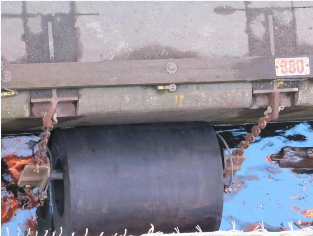
Figure 8. Cylindrical fender on Vanterm berth 5 (Source: TSB)
