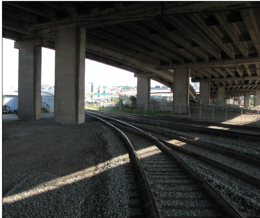
Photo 1. View to the west of the approach to turnout EL18
