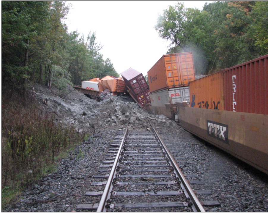
Photo 1. Clay on the tracks – looking westward
