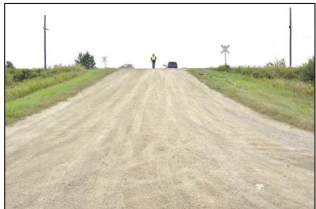
Photo 2. Southward view approaching the crossing from the north (12 August 2012)
