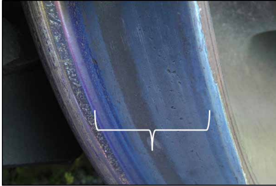
Photo 12. Blueing of locomotive wheel due to heat
