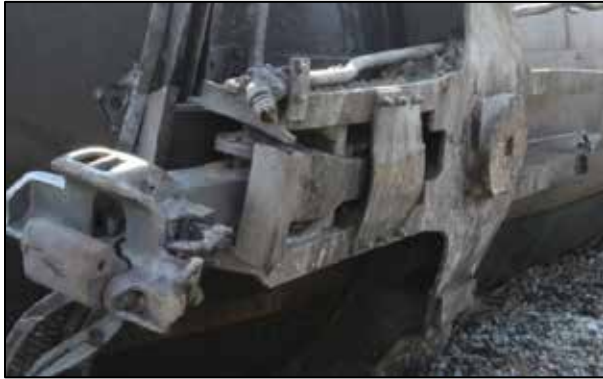
Photo 17. Complete stub sill
