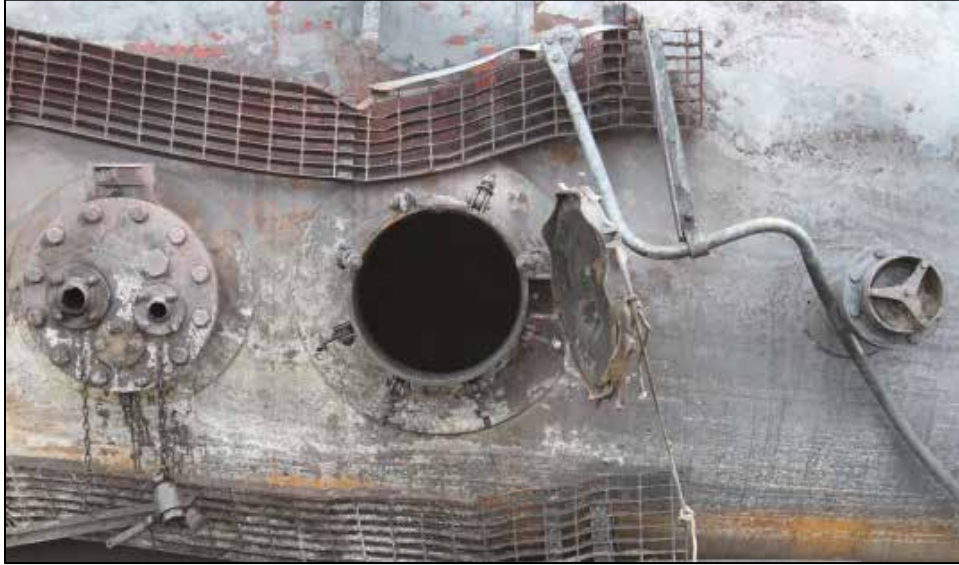
Photo 23. Manway cover and opening
