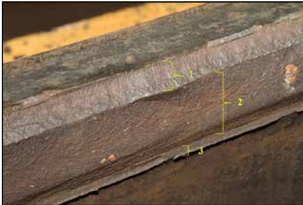
Figure 4. Close-up of gauge-side head fracture showing 3 zones
