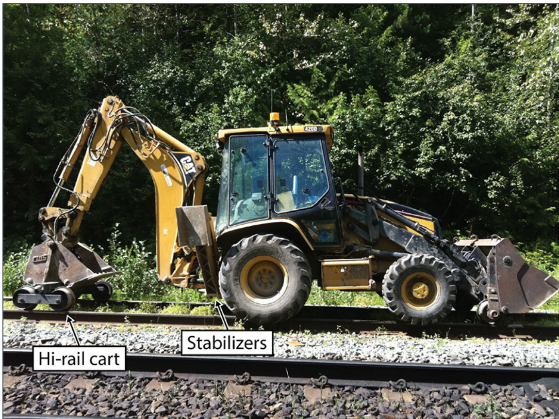
Figure 4. Similar backhoe with attached hi-rail-equipped cart
