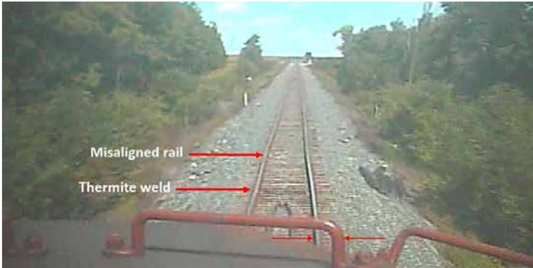
Figure 6. Slight rail misalignment just north of the thermite weld (Source: Canadian Pacific Railway, with TSB annotations)
